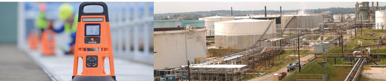
Tank farms are used to hold a wide range of products. In the headspace of each of the tanks within the farm, any number of toxic or combustible gases may be present. Radius BZ1 Area Monitors can be set up near a tank farm to make sure those toxic or combustible gases are not escaping into the environment.
